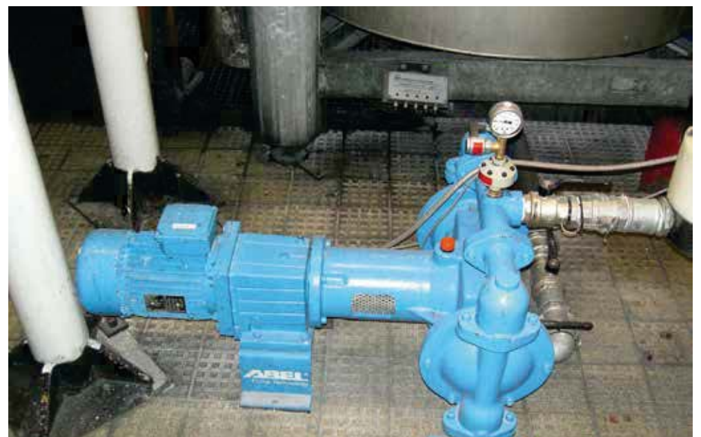
Electromechanical diaphragm pump, Type EM-040Z0300-SG as reflux pump for excess glue
